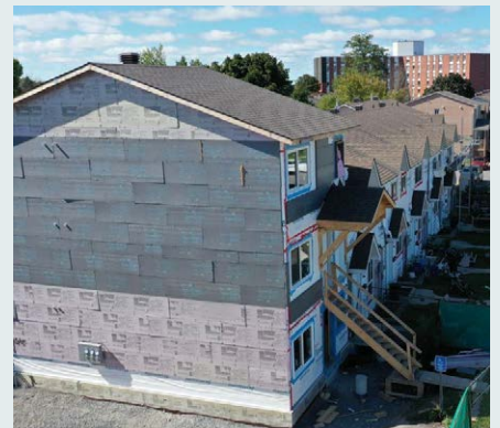
3. Exterior framing complete
