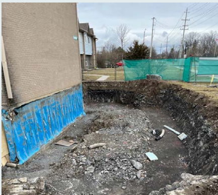
1. Excavation complete and ready for new foundations
