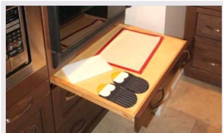
**Figure 13: A pullout shelf positioned below the oven can be used to place utensils or items that are going into the oven.**
