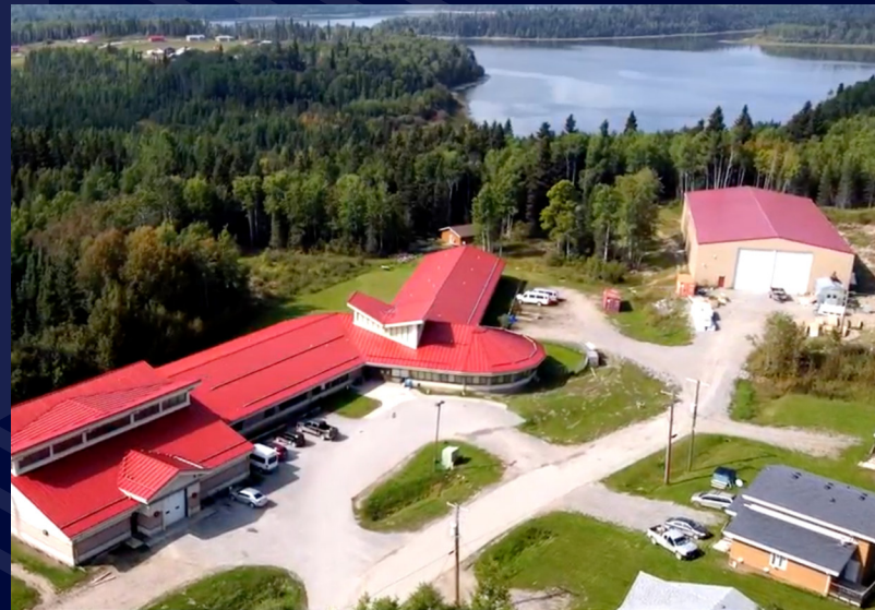
Pewapun Construction Ltd in Nelson House, Manitoba
