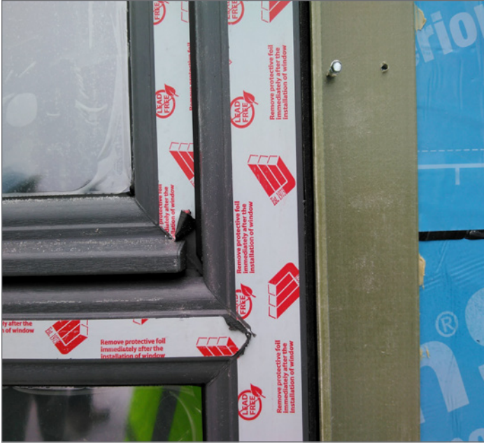
Figure 2 Window detailing for airtightness.
