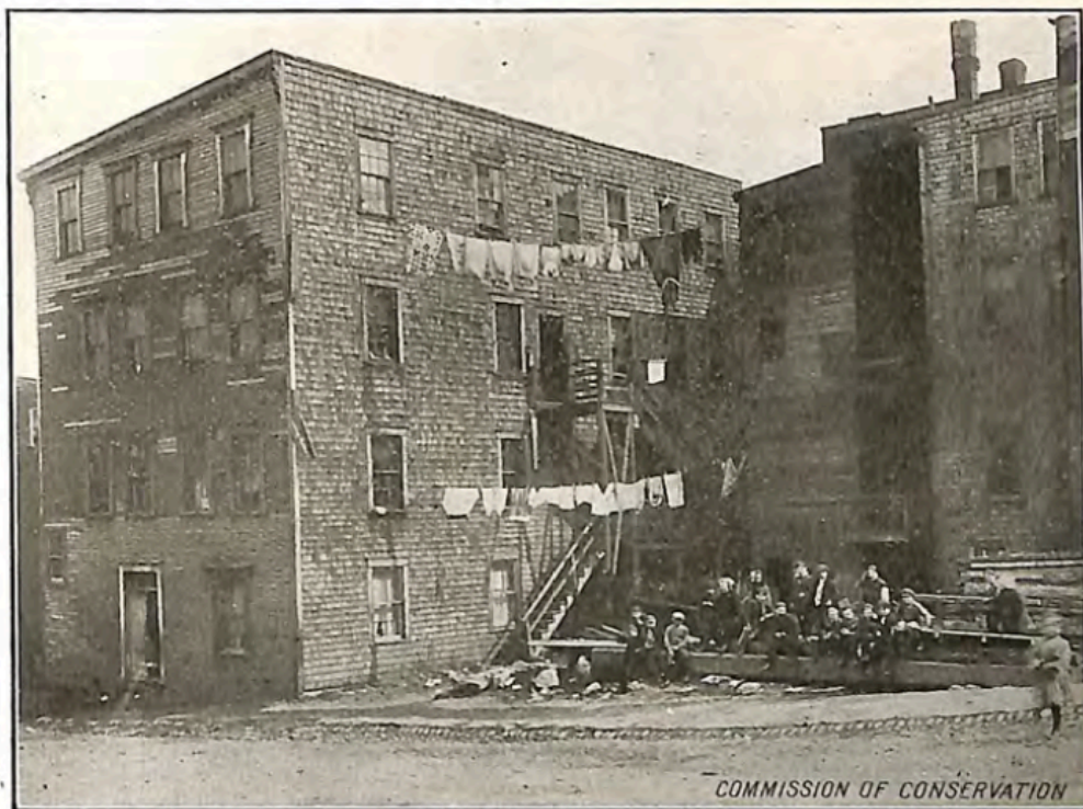
Four storey tenement house in a Canadian city occupied by eight families.
