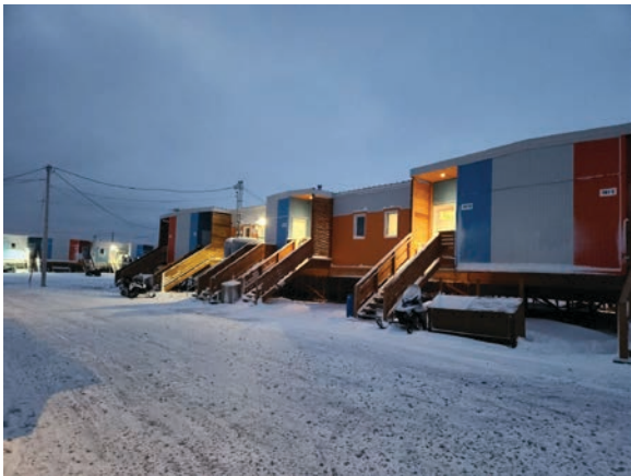
Sanirajak community housing, photograph, Bawating Building Science.
