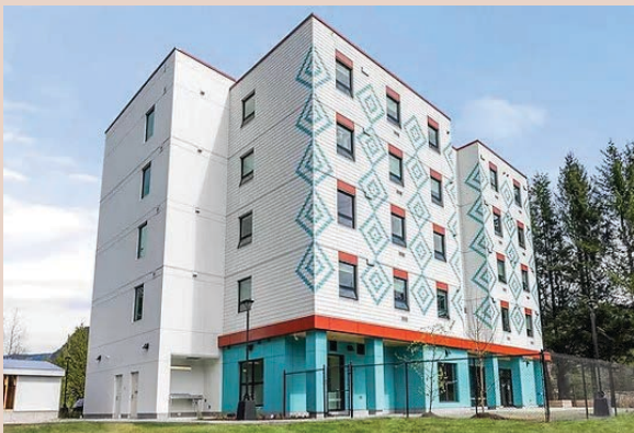
From top to bottom: Prefabricated modular unit installation, photograph; Estítkw Place exterior, photograph; Eskekexwi7ch tkl'a Sp'akw'us Place interior, photograph; and Eskekexwi7ch tkl'a Sp'akw'us Place exterior, photograph, NUQO Modular.
