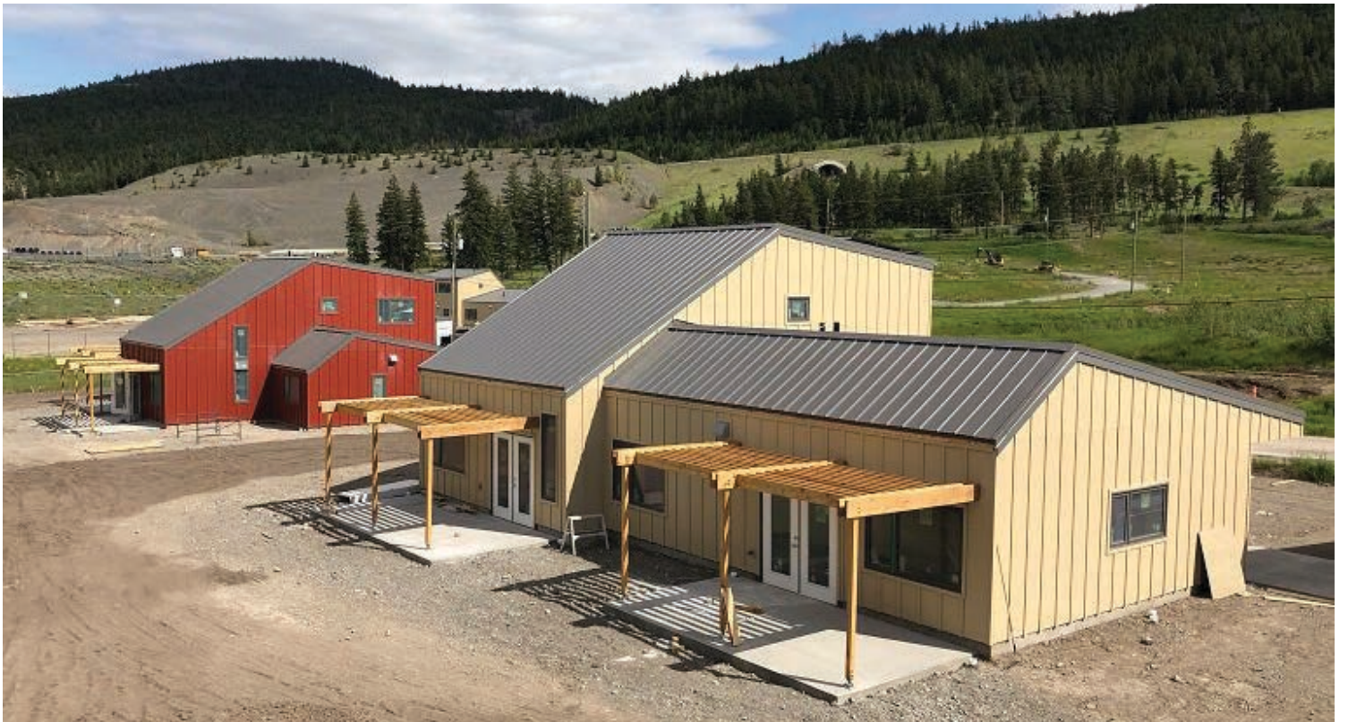
Three finished duplexes within the Cook's Ferry Indian Band community, photograph, Urban Arts Architecture.
