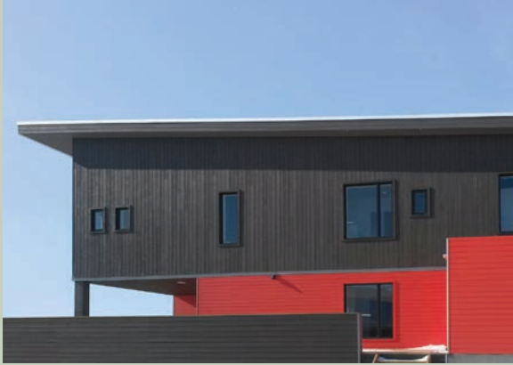
Supervised apartments façade, photograph, Blouin Orzes architectes.
