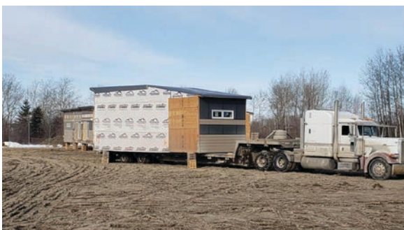
From top to bottom: Cardinal House cross-laminated insulated panel installation, photograph, Mark Hemmings; y-shaped Kivalliq Senior's Long-Term Care Facility, photograph, Verne Reimer Architecture Inc. and Blouin Orzes architectes; mass timber in the Wii Gyemsiga Siwilaawksat, photograph, hcma; and prefabricated units in the Pikangikum Safe House-Hotel, photograph, Grandeur Housing Ltd.
