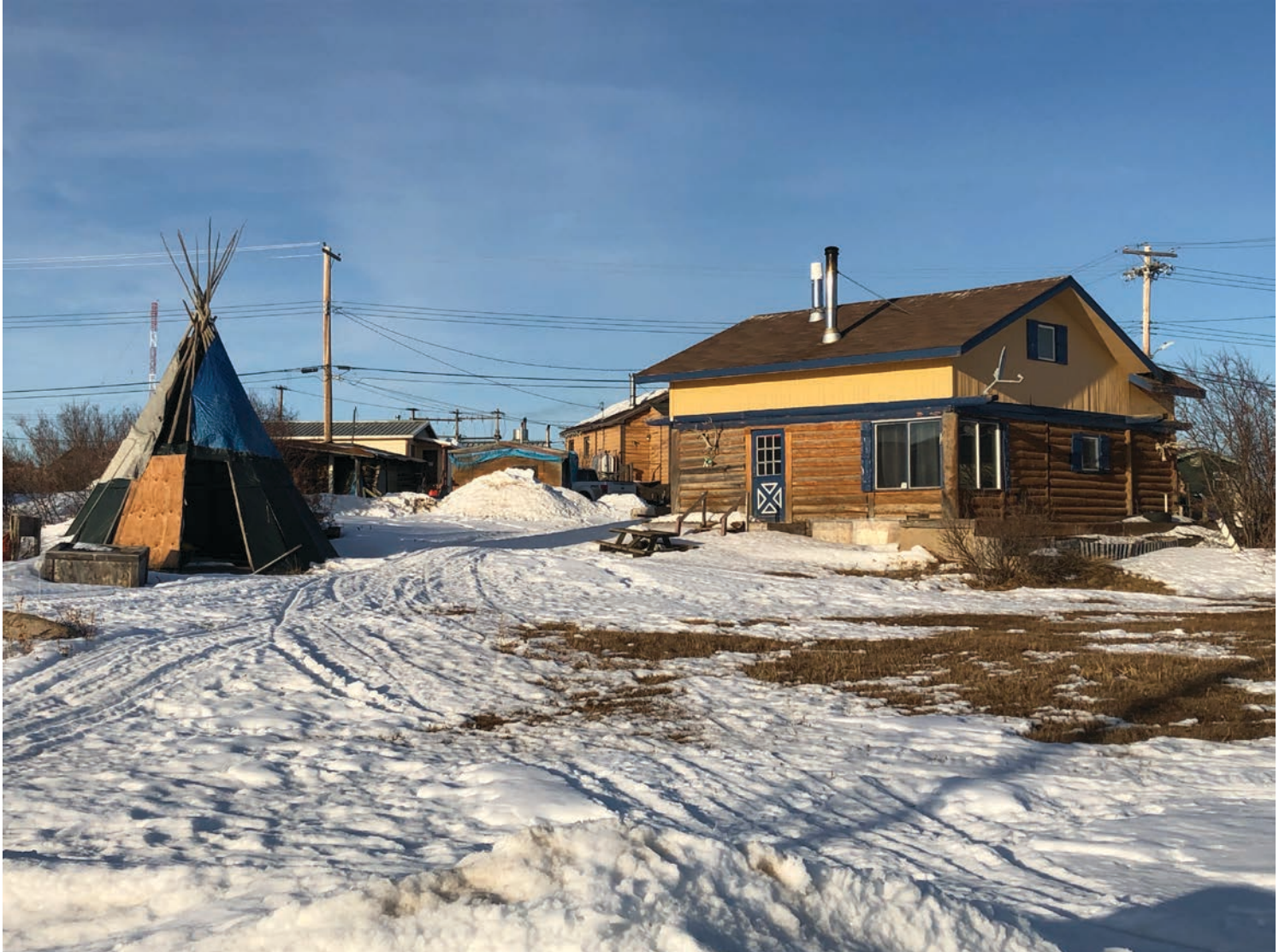
Délı̄nę community housing, photograph, Formline Architecture + Urbanism Inc., 2021.
