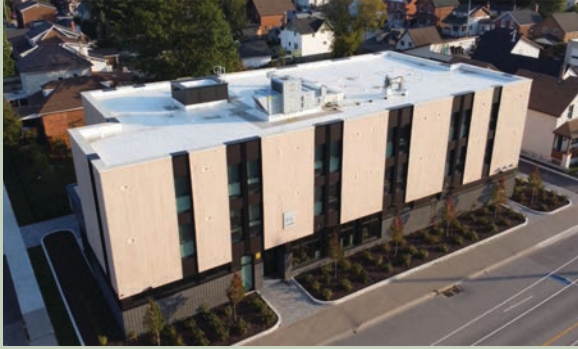
Aerial view, photograph, Designed Roofing.
