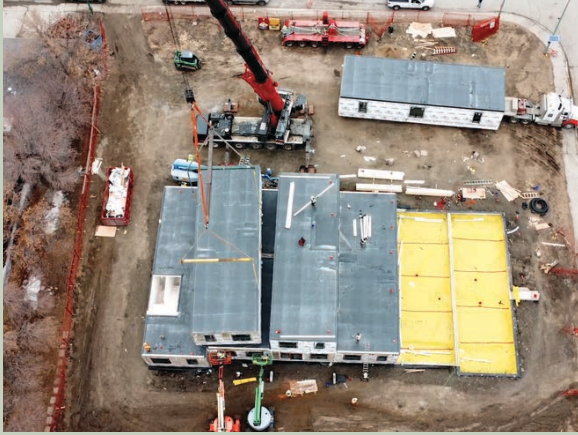
Modular units being craned into place, photograph, Big Block Construction.
