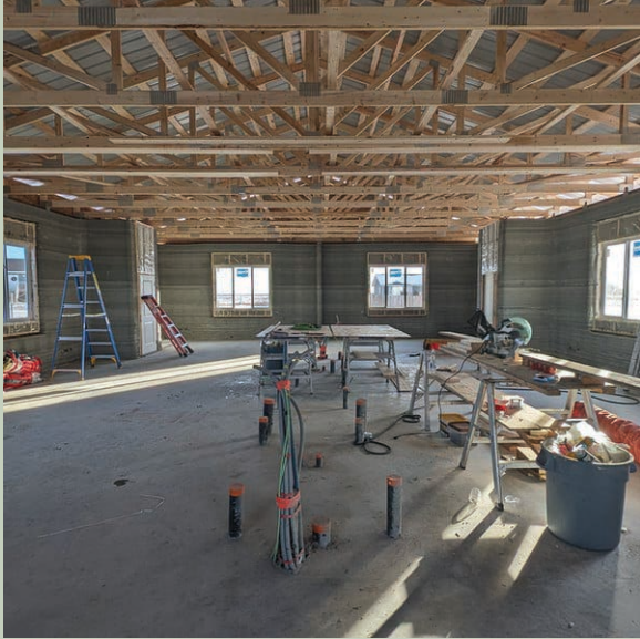
Concrete 3D printed home with roof framing installed, photograph, Siksika Nation Tribal Administration.
