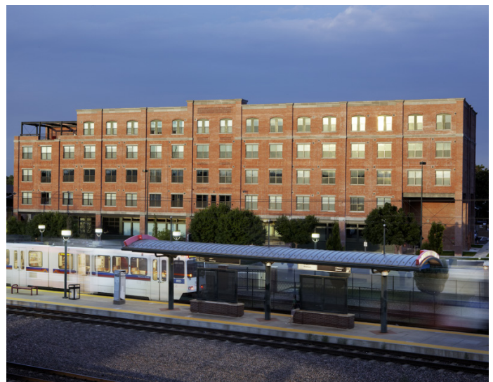
ULC funding redeveloped a historic building as the Evans Station Lofts, including 50 units of affordable housing next to the transit station.
