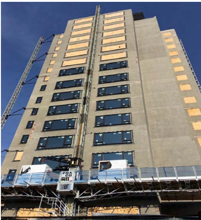
Figure 1: Ken Soble Tower renewal under construction, Hamilton, Ontario
