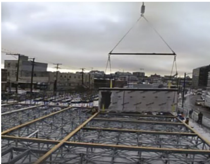
Figure 3: On-site construction phase—first modular unit lifted onto the movable foundation
