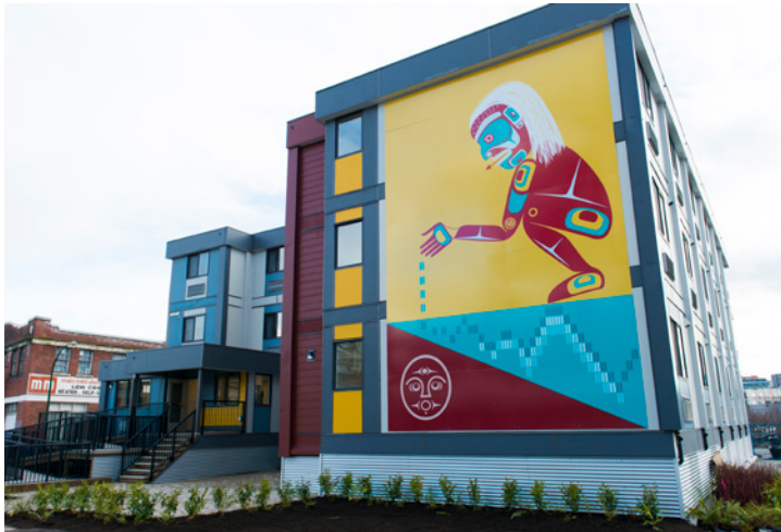
Figure 1: Front view of the 40-unit movable, modular building
