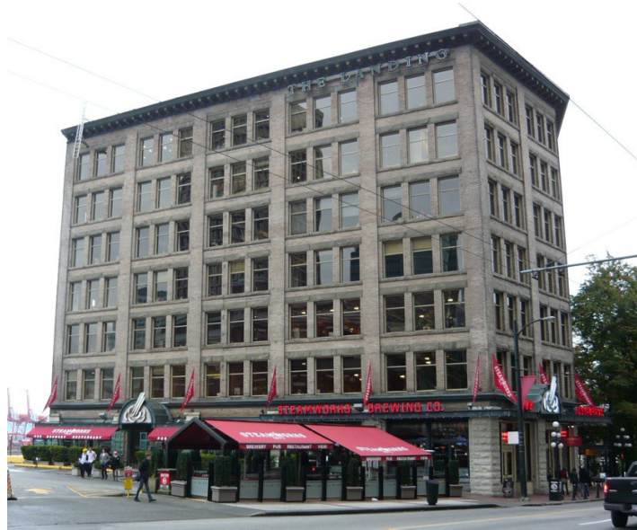
Figure 7. Vancouver’s first tall timber structure was the Kelly Douglas building (now known as The Landing) built in 1905 at 375 Water Street (Source: Canadian2006 , CC BY-SA 3.0 , via Wikimedia Commons ).
