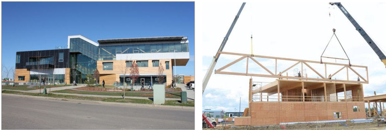
Figure 6. LEED Platinum Mosaic Centre, Edmonton, Alta. (courtesy of Mosaic Centre and Western Archrib).
