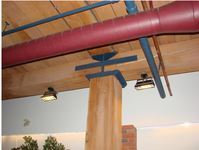
Figure 24. Connection in historical Leckie Building, Vancouver, B.C.
