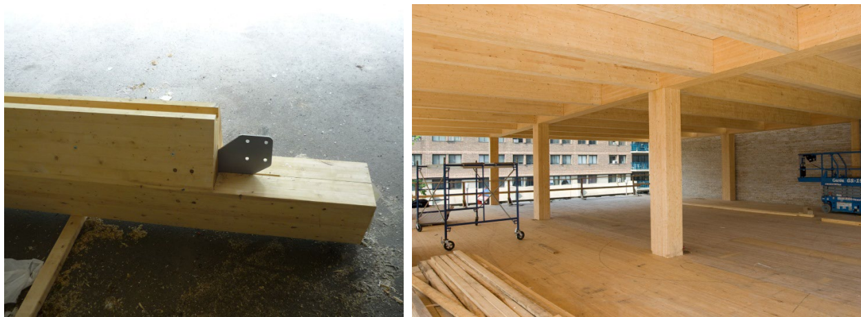
(a) Internal steel plate
