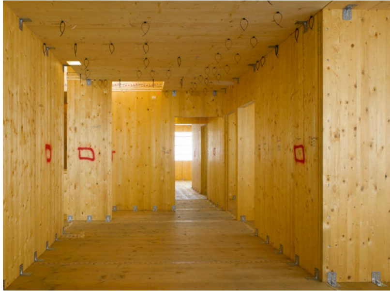
Figure 15. CLT panel structure (courtesy of Waugh Thistleton).
