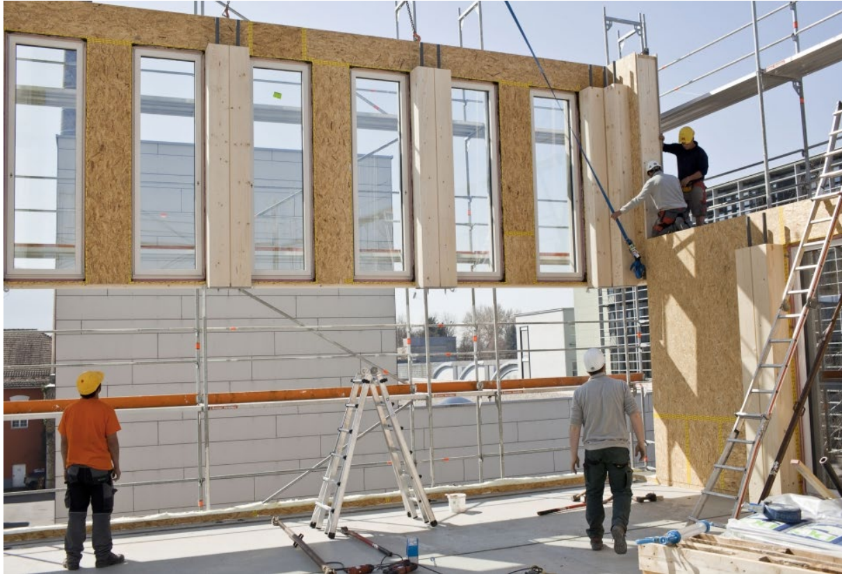
Figure 22. Facade panels (courtesy of CREE).
