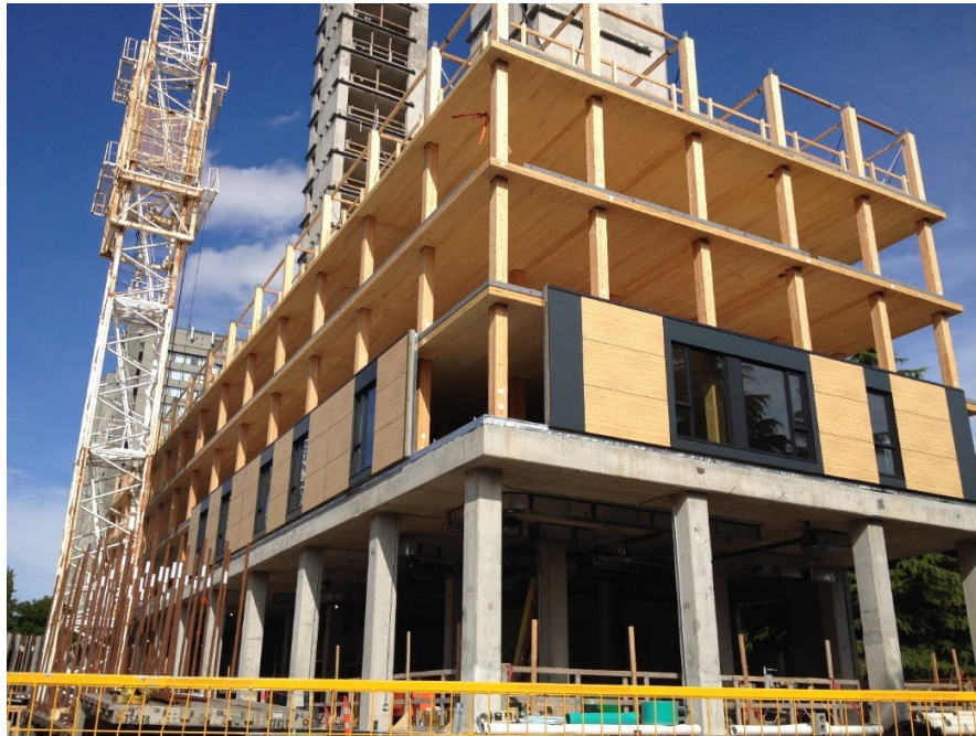
Figure 33. Concrete podium, UBC, Brock Commons (courtesy of www.naturallywood.com ).
