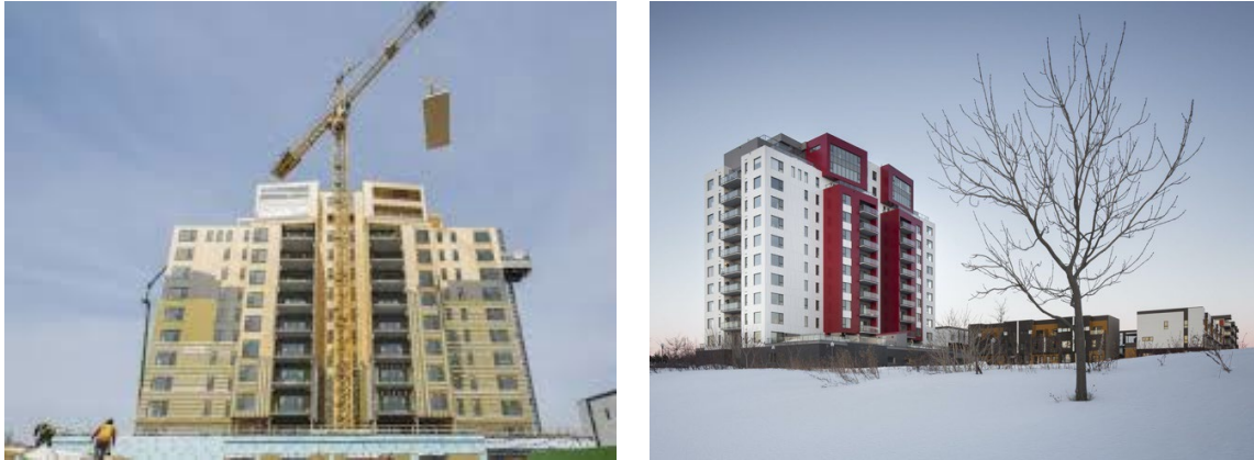
Figure 4. Origine apartment building in Québec City, fabricated out of CLT (courtesy of Cecobois).
