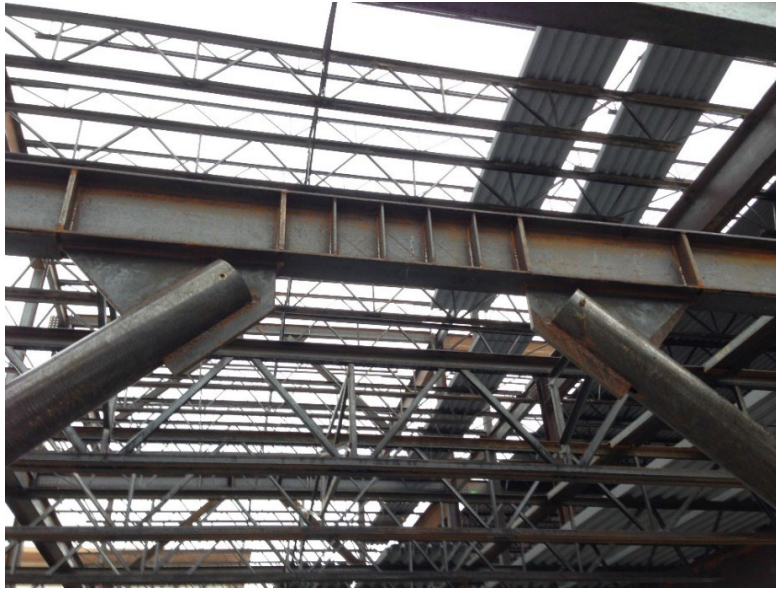
Figure 29. Steel EBF (courtesy of Andrew Seeton).
