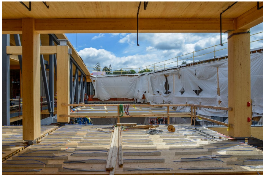
Figure 12. Timber-concrete composite slab system, University of Massachusetts, John W. Olver Building (courtesy of Alex Schreyer/ University of Massachusetts).
