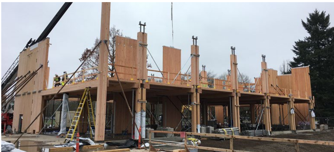
Figure 38. Erection of mass timber post-tensioned walls at the Peavy Hall building.
