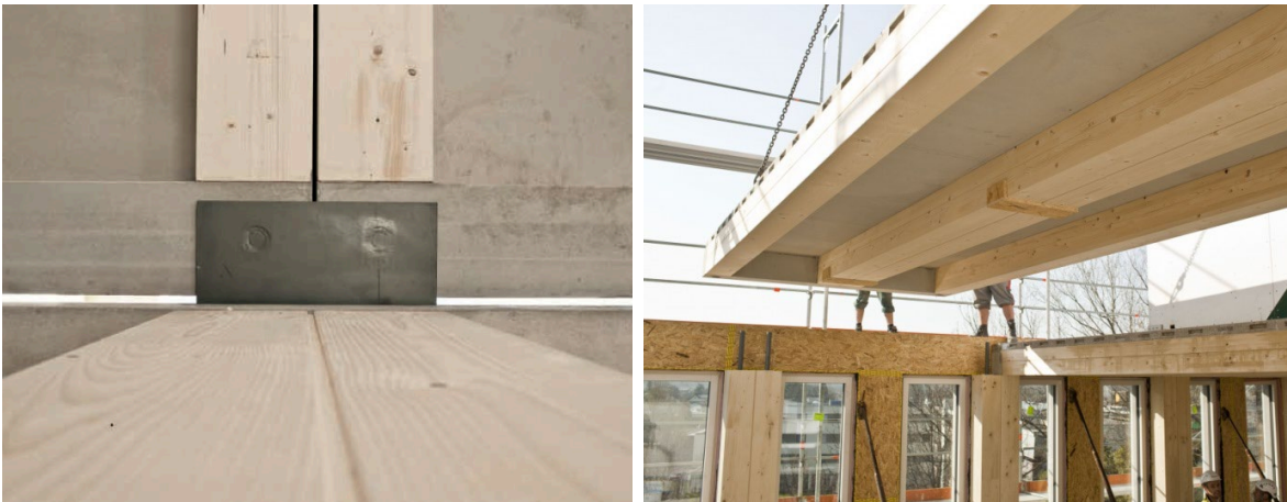
Figure 21. Column-to-slab connection (courtesy of CREE).
