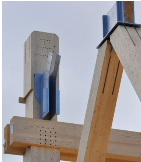
Figure 5. Brace and beam detailing, Synergia Complex, Saint Hyacinthe, Que. (courtesy of ©Nordic Structures).
