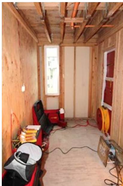
Figure 1. Air leakage testing of a single suite in a wood-frame multi-unit residential building (courtesy of RDH Building Science).
