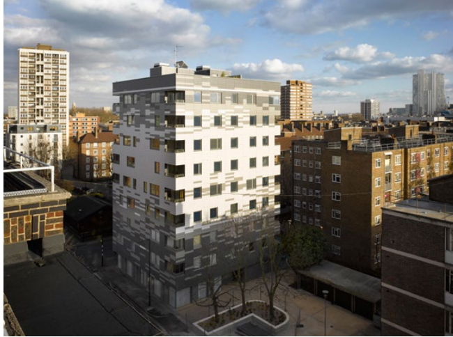
Figure 2. Stadthaus, London, UK (courtesy of Waugh Thistleton Architects).
