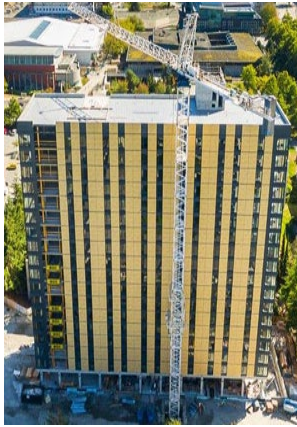
Brock Commons, Vancouver B.C. (18 storey)
