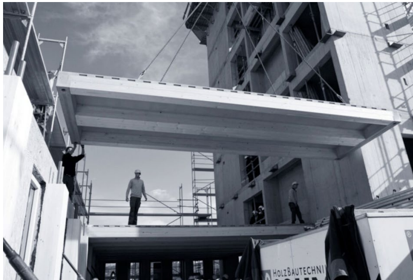
Figure 24. Floor slabs lifted into place (courtesy of CREE).
