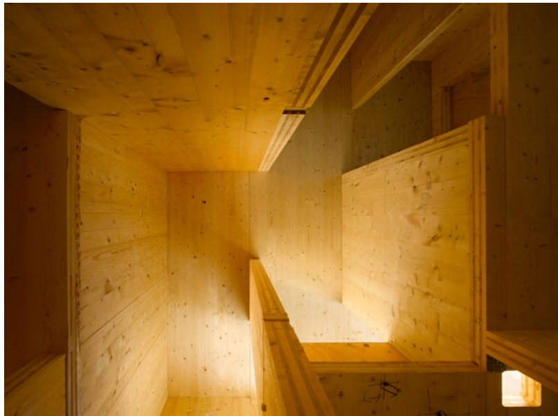
Figure 16. CLT panel structure (courtesy of Waugh Thistleton).
