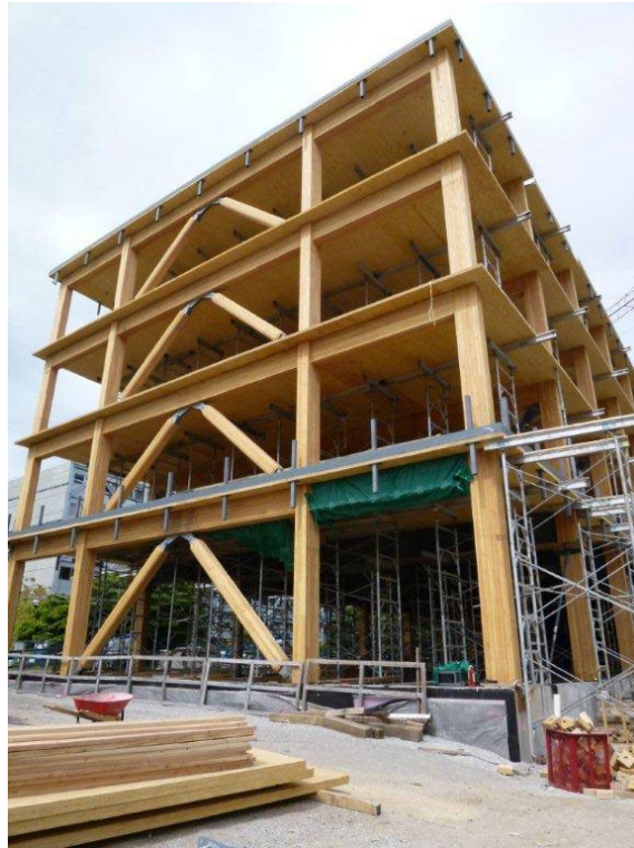
Figure 21. Braced frames, UBC, Earth Sciences Building (courtesy of Equilibrium Consulting).
