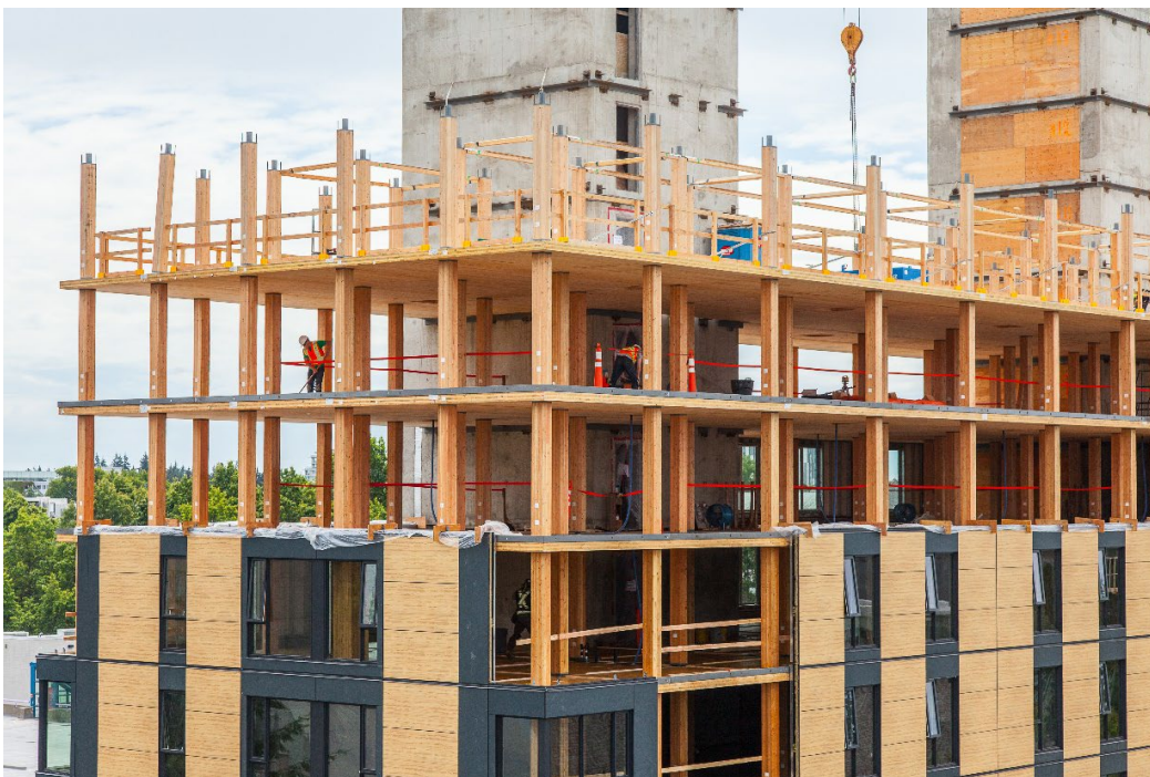
Figure 1. Point-supported CLT, UBC, Brock Commons (courtesy of www.naturallywood.com )
