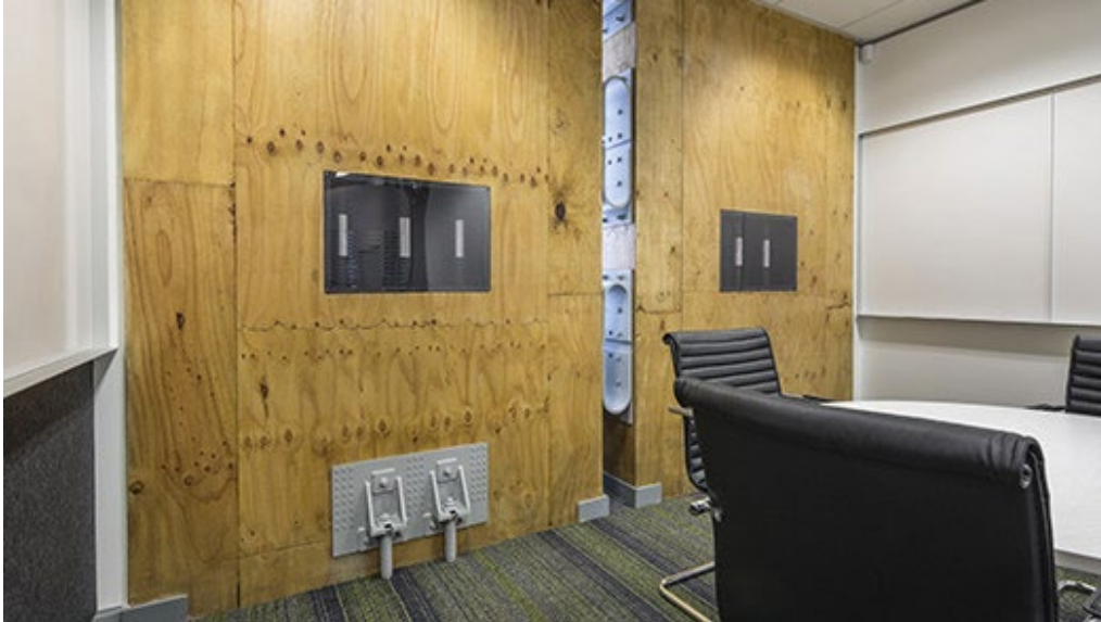
Figure 37. Coupled mass timber walls with post-tensioning cables and axial energy dissipators in the Trimble Office building, Christchurch, New Zealand.
