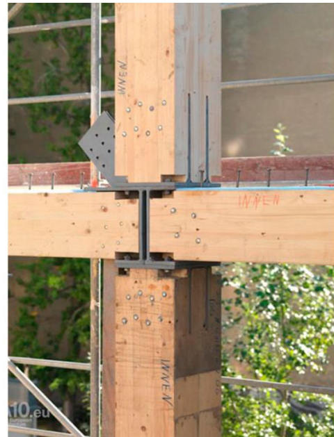
(b) 7-storey post-and-beam building, Berlin
