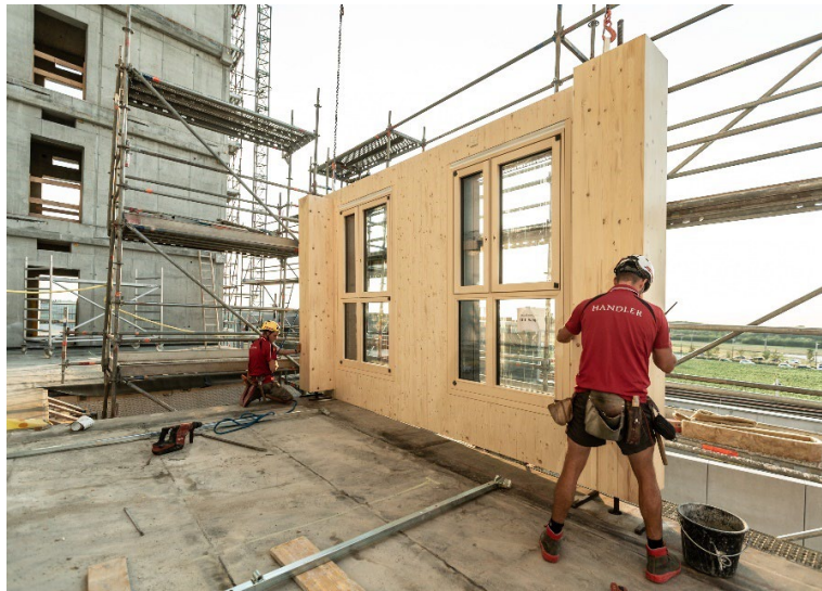
Figure 15. Prefabricated panel installation, HoHo (courtesy of cetus Baudevelopment + Thomas Lerch).
