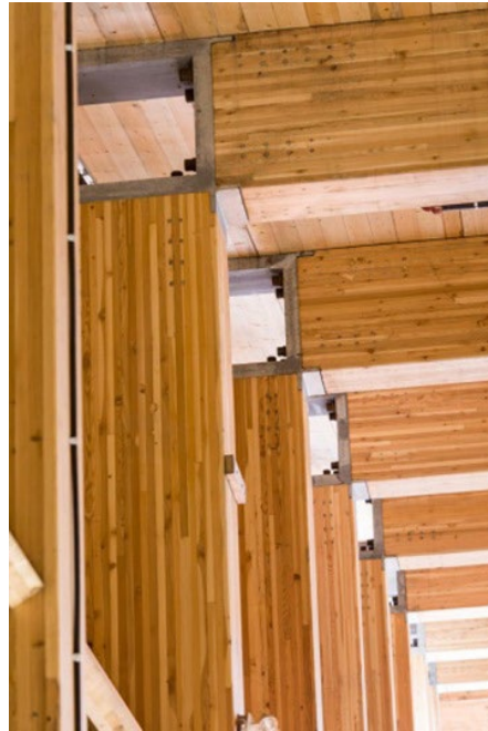
Figure 22. Moment connection, UBC, Bioenergy Research Demonstration Facility (courtesy of Don Erhardt).
