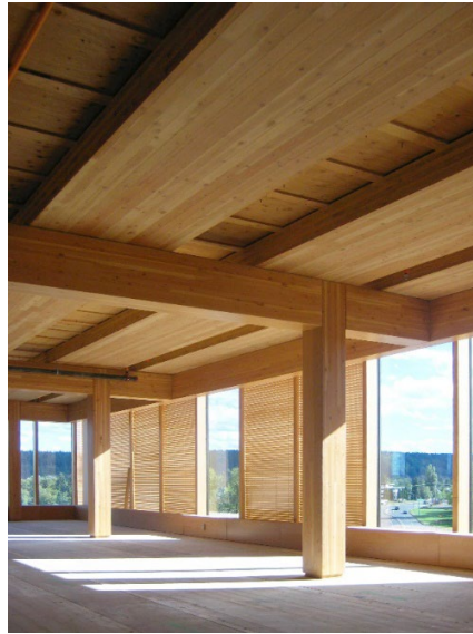
Figure 8. Posts and beams, Wood Innovation Design Centre (courtesy of MGA | Michael Green Architecture).
