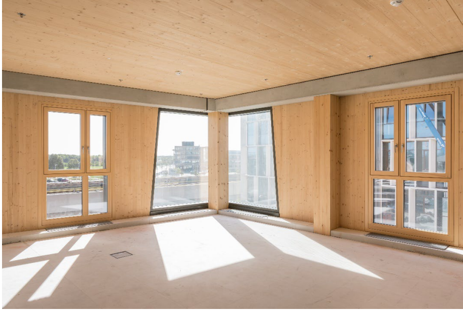
Figure 26. Interior of exposed timber structure (courtesy of Cetus Baudevelopment).
