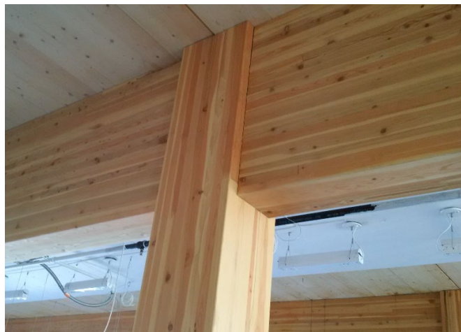
Figure 9. Concealed beam to girder connections.
