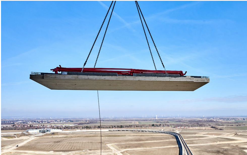
Figure 25. Floor panels with preinstalled services (courtesy of Cetus Baudevelopment).
