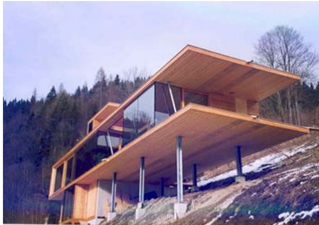
Figure 10. Massive-wood floor plate on posts where punching shear is likely to govern design (courtesy of KLH).
