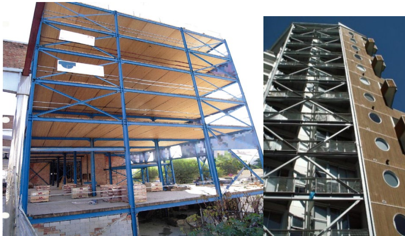
Figure 27. Steel-timber hybrid, Spain (left); Scotia Place, New Zealand (right).
