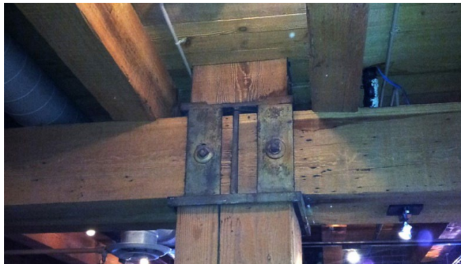
(a) Historical building, North America
