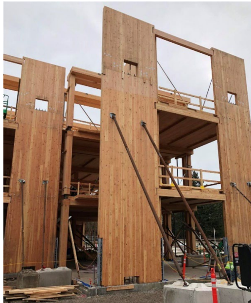
Figure 24. Post-tensioned shearwall, Oregon State University, Peavy Hall (courtesy of Equilibrium Consulting).
