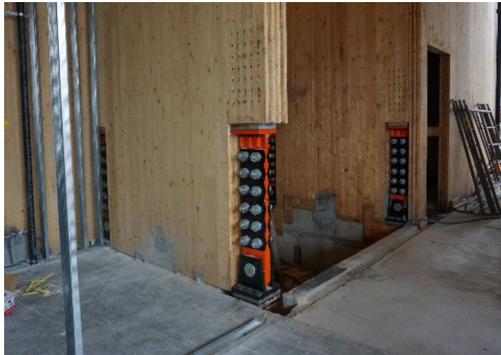
Figure 31. Tectonus resilient slip friction joint used as shearwall hold-down (courtesy of Fast + Epp).
